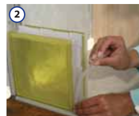
2 Mount the short seal profiles to the sides.
