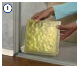
1 Assemble the frame profile and insert the first X-BLOCK.
