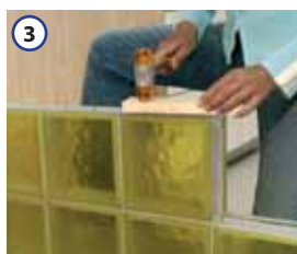
3 Mount the long seal profiles onto each complete row.
